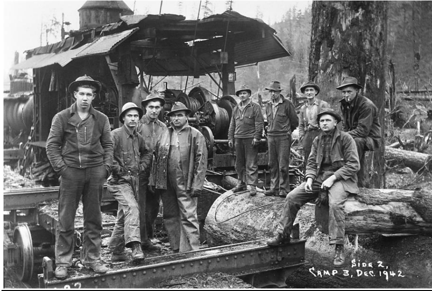
Yarding Operation with a steam driven “Donkey” engine in the background photo courtesy of Kaatsa Station Museum & Archives KSM-A-N00893-nd-NIS
