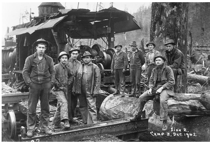
Yarding Operation with a steam driven “Donkey” engine in the background
